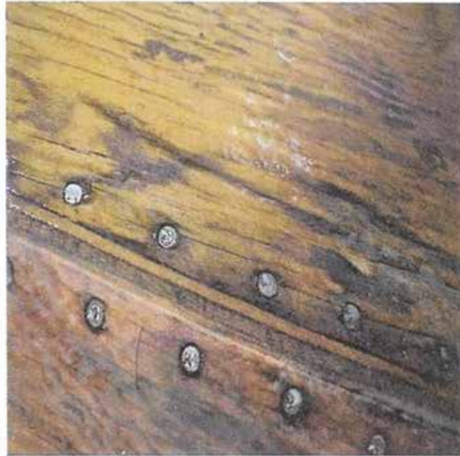
Stainless steel Anchorfast nails. Anchors on every one.
